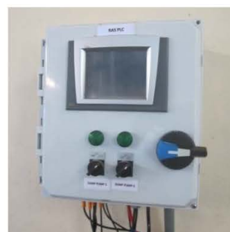
Programmable Logic Controller of the RAS
