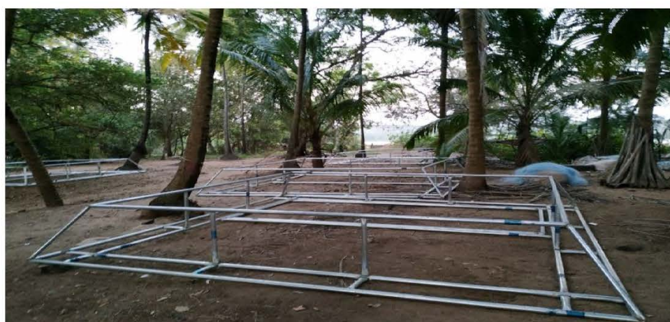
Welded cage frames
